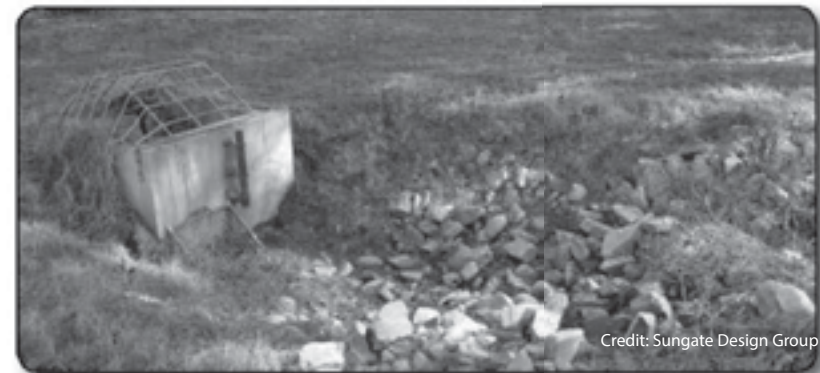
This existing stormwater control structure at the I-440/Wade Avenue interchange controls runoff rates.
